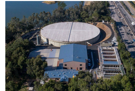
Montevina Water Treatment Plant
